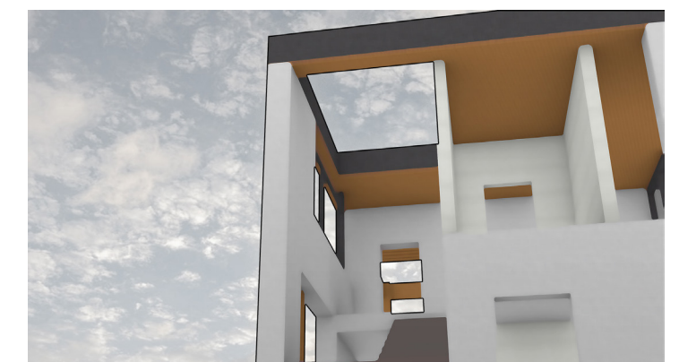
Roof skylight makes the vertical massing even more transparent.
